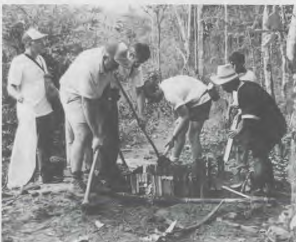
At the worksite, ADRA volunteers and local residents break the ground where water pipe will be laid.
