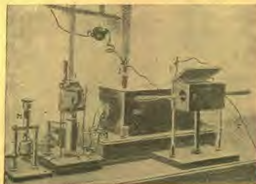
The Sending Instrument of a Wireless Telegraph Station. M is the Sending Key; I, the Motor Driving the Interrupter of the Coil; B, Pt, the Connection with the Mast; O, the Oscillator; and i, the Connection with the Earth.
