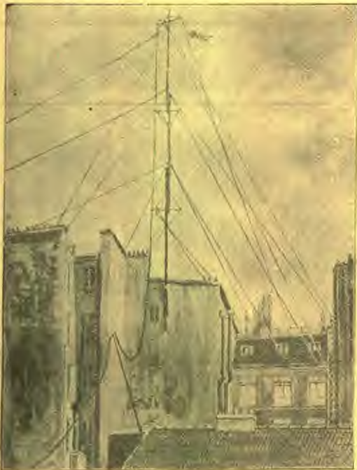
The Mast of a Wireless Telegraph Station Carrying the Wire Called the "Vertical Conductor," from which the Messages Leap off into Space.
