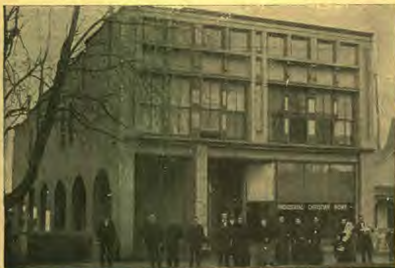
The Industrial Christian Home, Ogden, Utah.—Front View.
