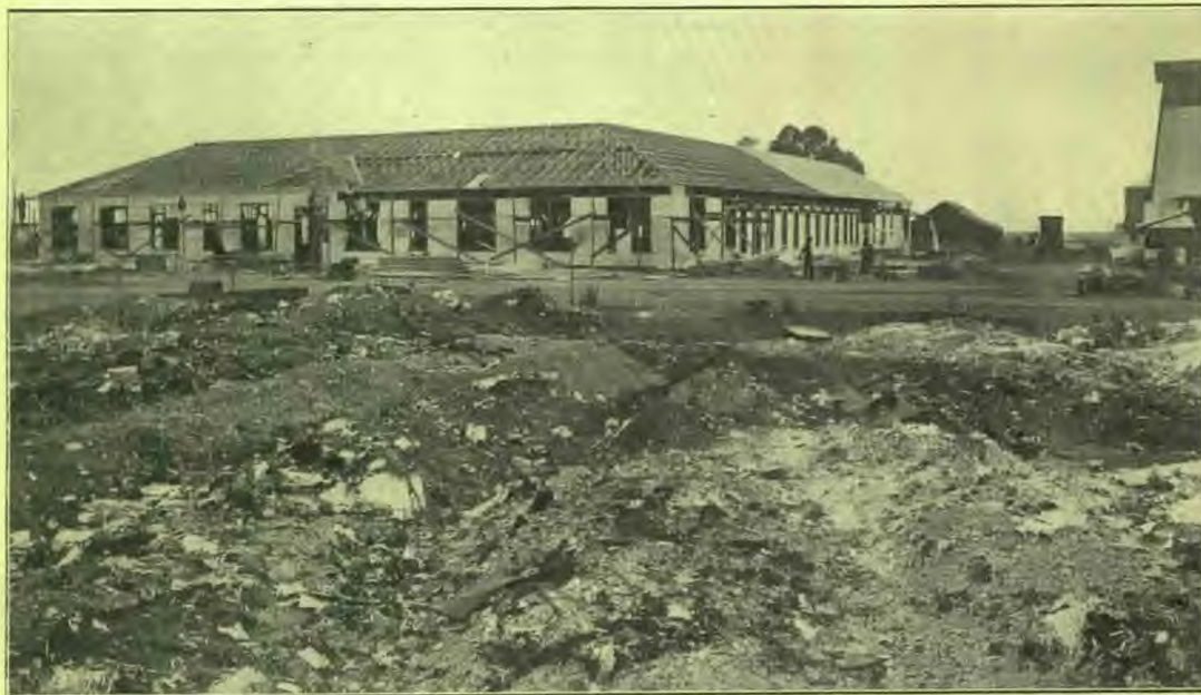
Pacific Press Building Dec. 7, 1906. In the foreground are the heaps of ashes and debris removed from the burned building. The photographer, Mr. F. H. Gage, placed on the photo this legend: "From the ashes of the old, the new building is arising." It is much farther advanced now than when this view was taken. All who see it pronounce it an economical, model factory building.
