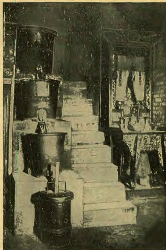
Old Water Clock, Canton, Flow of Water from Bronze Tank to next Is so Regulated that the Rise on the Graduated Rule Indicates Time of Day.
