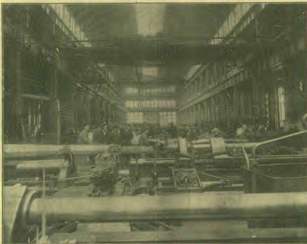
Gun shop of the Navy Yard, Washington, D. C. The cut shows the monster traveling cranes overhead that can pick up any of those large guns and place them in whatever position may be desired by the workmen. It also shows the work of turning and boring the guns.
