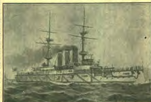
Japanese battle-ship "Shikishima." Displacement, 15,000 tons. Speed, 18 knots. Guns: 4 12-inch; 14 6-inch; 20 12-pounders, and 8 3-pounders.
