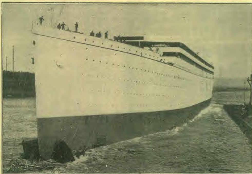
The " Olympic " of the White Star line just after she was launched. Note the five lower decks and four upper ones. The rudder of the ship alone weighs 100 tons. There are 2,500,000 rivets in the boat. Each engine crank-shaft weighs 118 tons. Anchors weigh over 15 tons, and each link of their cable chain weighs several hundredweight. She is simply a mammoth. In 1811 there was built in Nord's yard, at Port Glasgow, the famous Comet of 25 tons. In 1911 the Olympic , of 45,500 tons, sails from Liverpool; and the Cunards Company , we are told, will follow with one 500 tons larger.
