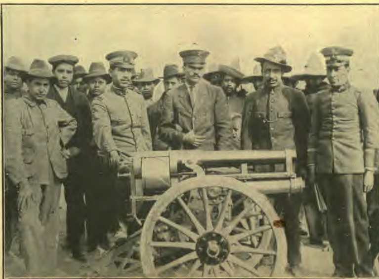
The revolver cannon, invented by E. Duron, a Mexican colonel. It can shoot thirty four-inch shells a minute. It can be disassembled readily, and can be conveniently moved about, weighing only seven hundred pounds.
