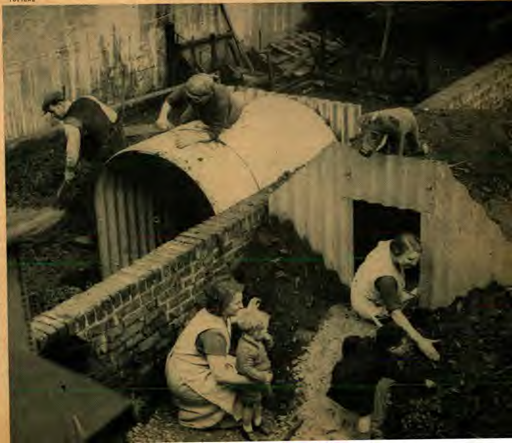
Homes of the future in London. Government-provided steel air-raid shelters being erected in the little back yards of the Borough of Islington.
