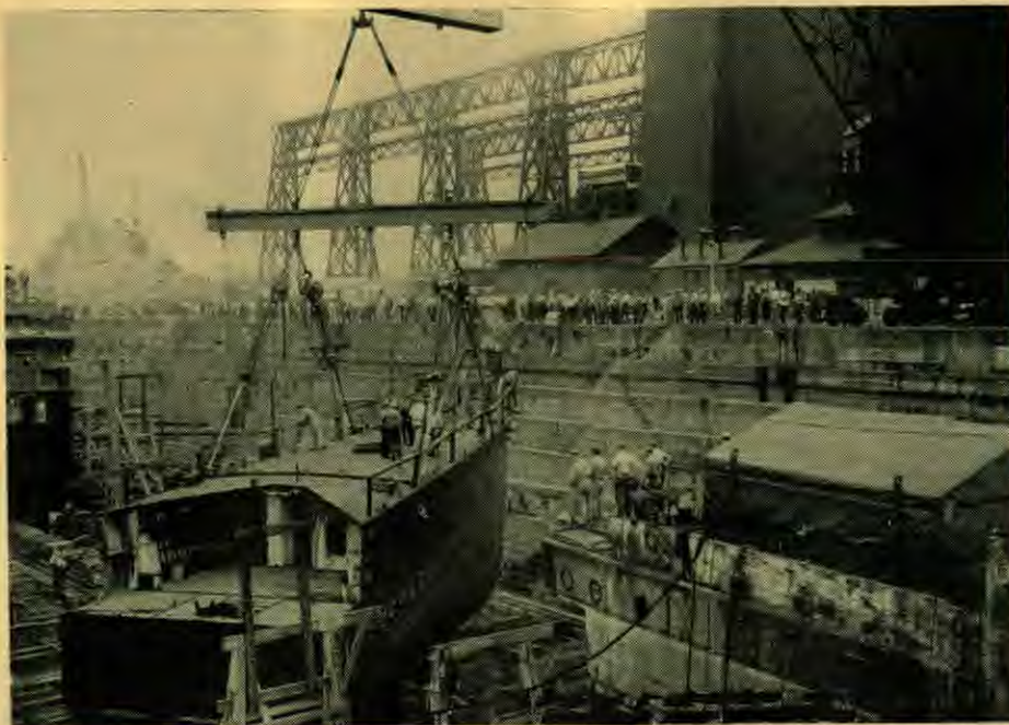
The bow of a decommissioned destroyer is here seen in process of being transferred to another ship whose bow was wrecked by a torpedo in the Caribbean Sea.
