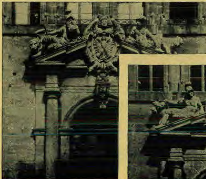
Carved in stone in 1607, these figures above the doorways of Nuremberg's ancient city hall portray the four beasts of the prophecy of Daniel 7. Though the hall was severely damaged during World War II, the carvings remained, mute illustration of the permanence of inspired prophecy.
