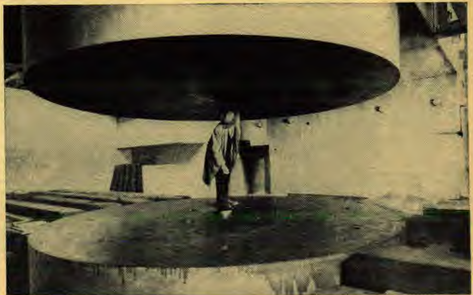
An inspector checks the huge 82-ton all-steel disks which will form the magnetic heart of the University of Chicago's new atom-smashing machine.
