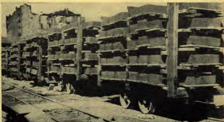
In Warsaw and other ruined cities of Europe, rubble is being made into cement blocks for use in rebuilding. Special mills are located in the devastated areas where the rubble is ground and mixed with cement.
