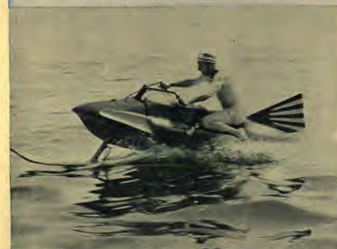
A new approach to water skiing is demonstrated by a man riding the "Chaffee-Ski," a watery version of a motor scooter. The craft mounts on two separate in-line skis with a 25 horsepower outboard motor mounted between them. The scooter is capable of speeds up to 50 mph. The sport bids fair to become popular.
