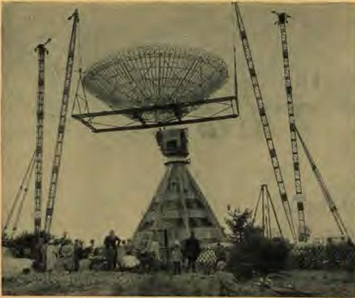
Two giant cranes lift the 80-foot-wide parabolic antenna onto the pyramidlike concrete base of the new radio-telescope of the Bonn University in Germany. It will be used for astronomical research.
