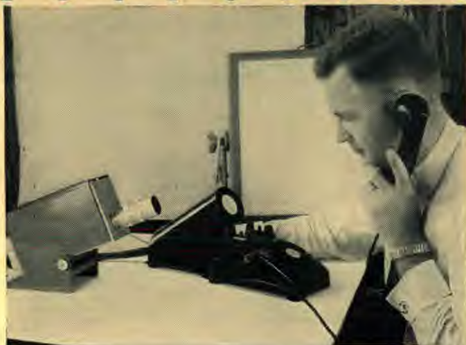
An engineer at the Bell Telephone Laboratories in New York demonstrates how the experimental picture-phone system operates. A picture of the party at the other end of the line is transmitted on the small oval attachment on the phone while the camera unit transmits a picture of the person who has dialed.
