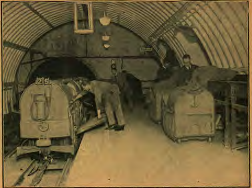
Sport & General Photo A miniature "tube" railway, 6\frac{1}{2} miles long, for the London postal service, was recently completed at a cost of £1,500,000. The trains, which are driverless, run on a 2-foot gauge double track laid in one tunnel of 9-foot diameter. This service is the first of its kind in the world.
