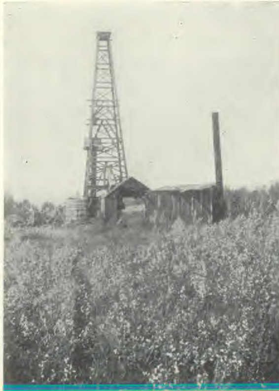
This photograph of an oil derrick will be very familiar to all who have visited oil field operations. The standard derrick is 72 feet high.
