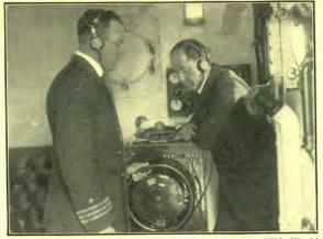
The mechanism shown in this illustration is the hydrophone which was perfected just before the signing of the Armistice. This instrument is for protection of ships in fogs, collision, and battle. It enables a pilot to calculate the distance of other ships and their speed, also the location of rocks, and the depth of the water.
