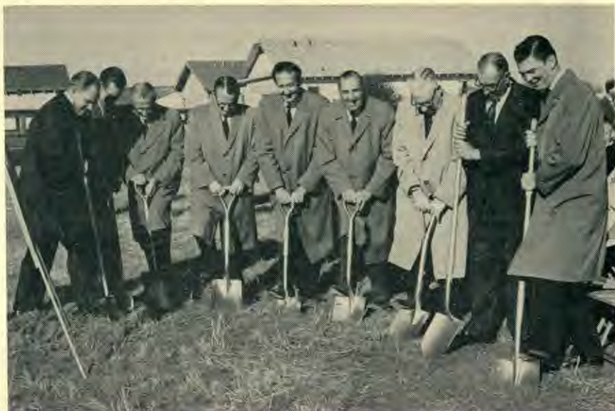
Groundbreaking ceremonies for a new church building for the Hemphill Seventh-day Adventist Church were held on Sunday afternoon, November 29, at the future building site on 2900 South Freeway, Fort Worth, Texas. The contemporary design building will have a seating capacity of more than 1100, and will provide for an evangelistic center. Elder W. R. May, pastor, Elder B. E. Leach, President of the Texas Conference, and Claude Dortch, chairman of the building committees, turn the first spades of soil.
