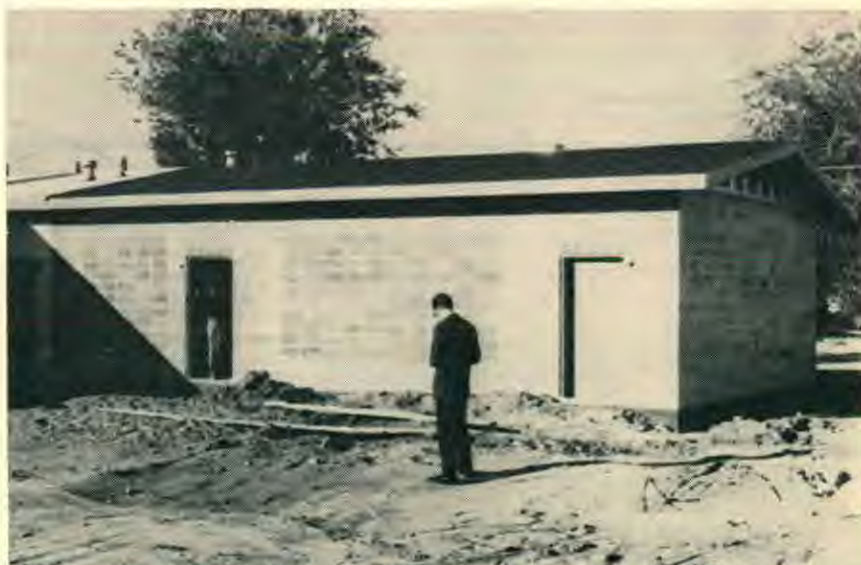
A new face is emerging in the Rocket City, Alamogordo, New Mexico. Pictured is what soon will become added school rooms and recreational facilities of the Seventh-day Adventist Church. Local elder J. O. Beucler is leading out in this $6,000 church addition project. H. W. Pritchard.
