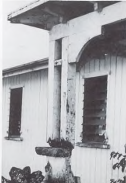
A decaying section of one of the several makeshift buildings which at present serve as dormitory accommodations for the young men at Fulton College, Fiji. The existing dormitories were originally built in the days of the Second World War from used materials.
