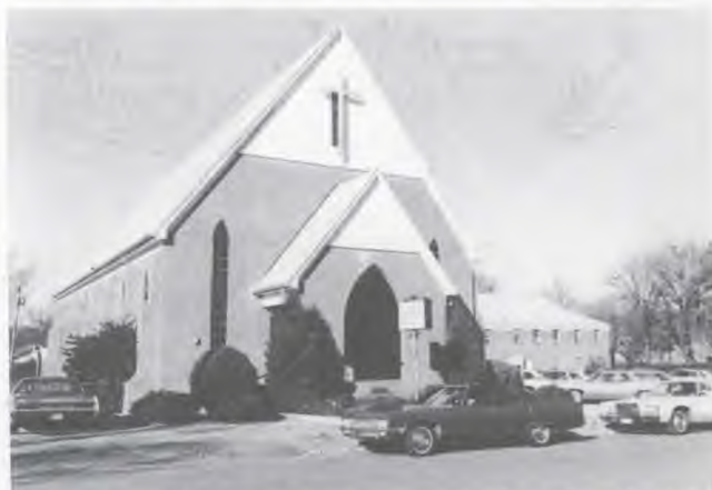
New Little Rock church and educational building opened December, 1975
