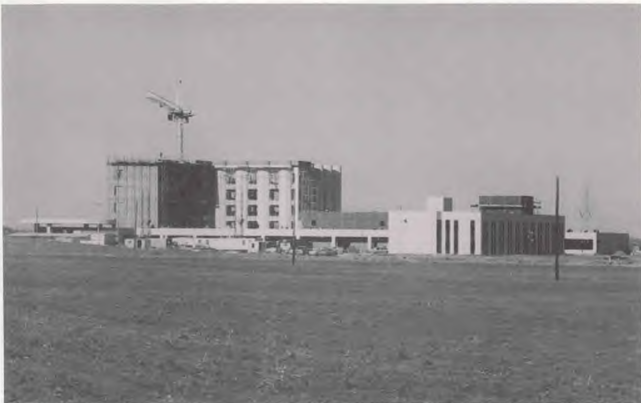
Huguley Hospital complex under construction
