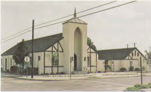
1 An attractive and comfortable church home in Lubbock, Texas. This church was partially destroyed by tornado and restored to service.
