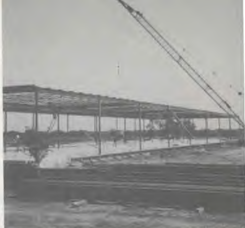
Pictured here is construction of the new Professional Building for Memorial Hospital, at Beeville. It will house 14 physicians. Cost will run $800,000.00 for the 27,000-square-foot building. It has been funded by community gifts. Completion is set for October, 1977.
