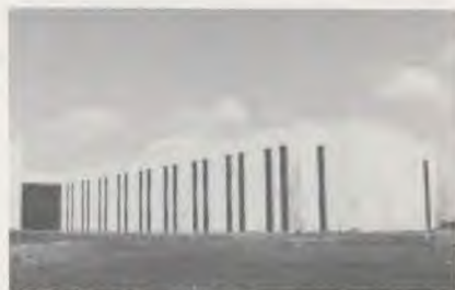
The Huguley Medical Office which eventually will contain 18-20 suites.
