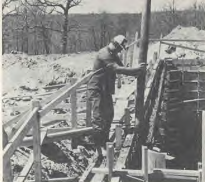
Stanley Buckmaster guides the cement into the side-wall form.
