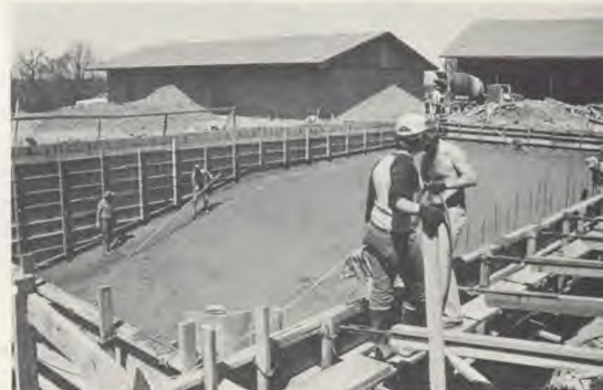
Finishing the surface of the cement on the pool floor required much careful work. In the background are the bath house, left, and the lodge.
