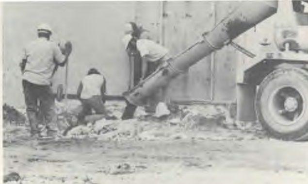
Workmen pour foundation for doctors' offices addition.
