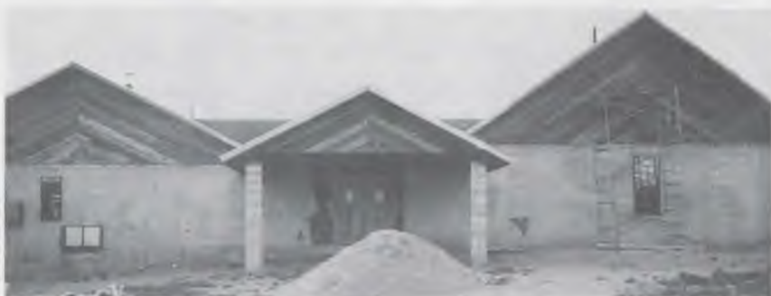
TEXICO EXPANSION FUNDS AT WORK — Construction is going forward on the Santa Fe English church. A portion of Texico Expansion funds is used for building new churches.
