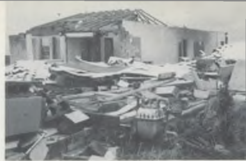
The remains of the Saragosa Church School building, which was not in use at the time.
