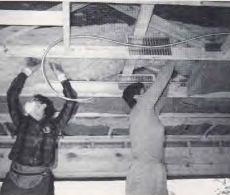
The ladies as they put up the insulation.
