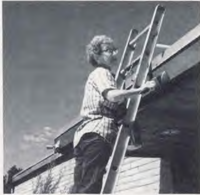
Not only did Maranatha help in the building of the cafeteria, but they painted and repaired other buildings on the Sandia View grounds.
