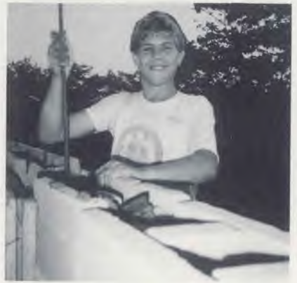
Jason Perkins filling concrete blocks for reinforcement.
