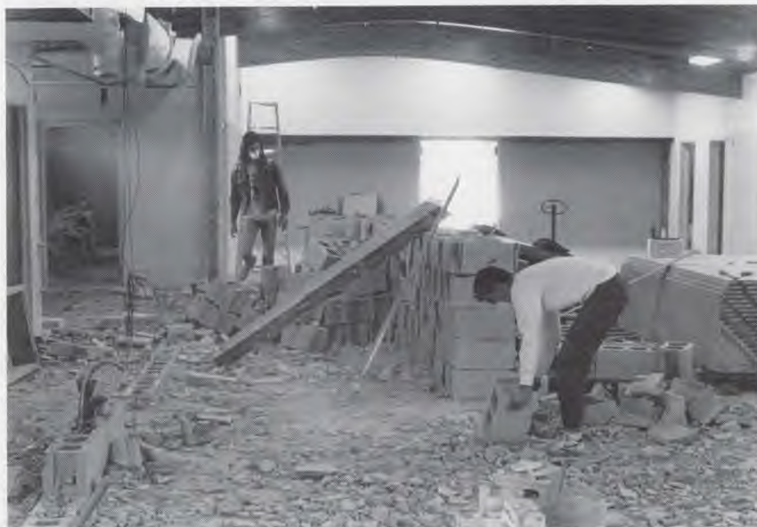
SAC students assist in converting the old ABC building into the new nursing department facilities.
