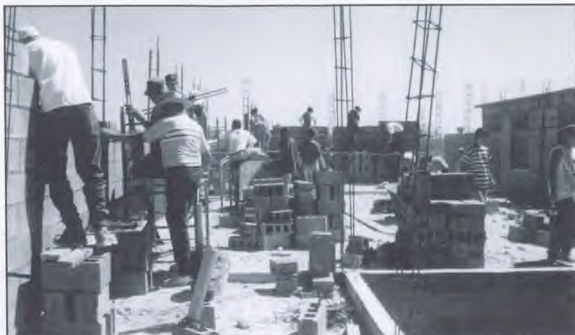
Students and sponsors in action at the building site in Miguel Aleman, Mexico.
