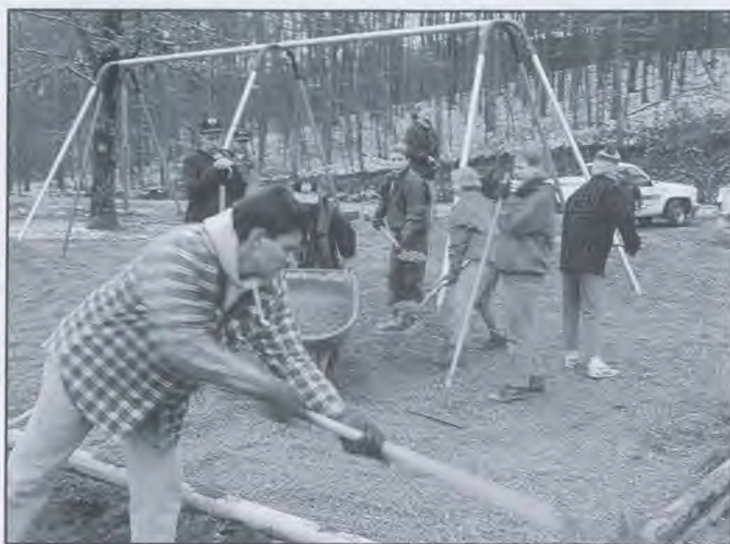
Pathfinders, putting into action the theme of "Making A Difference," spread gravel around a swing set in the National Park in Hot Springs, Arkansas. Photo: Michael Edge
