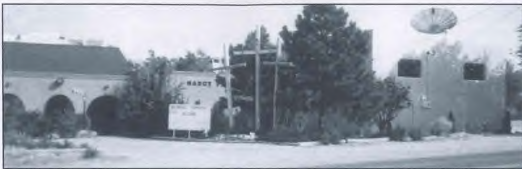
Thanks to Santa Fe Marcy Park volunteers under the leadership of former pastor Walter Vhymeister, Joe Gallegos, and Mr. and Mrs. Lonnie Smythe, a new gymnasium with a new satellite dish to the right of the church was completed. This will enable groups to receive messages from the General Conference and 3ABN. Photo: Peter Weber
