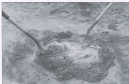
Backbreaking work—mixing cement by hand.
