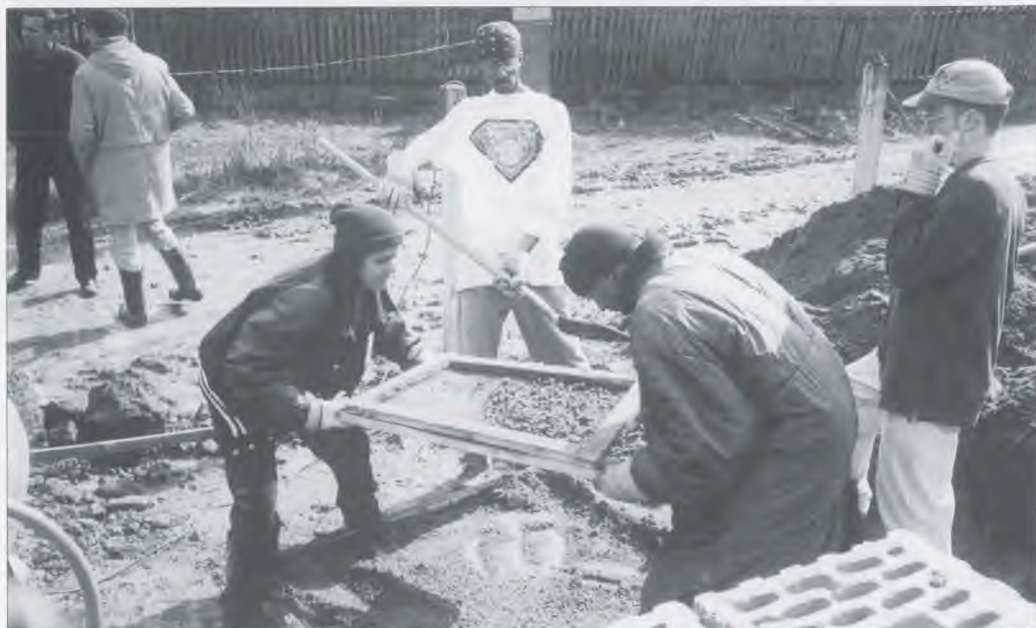
Mission trip members (l-r) Nadia Sarria, SWAU; Jason Moses, Burton Adventist Academy; Jermicah Jordan, Burton Adventist Academy; and Tom Lemon, SWAU, sift sand gathered from nearby riverbanks to mix with cement to create mortar for the walls of a church in Sovata, Romania.
