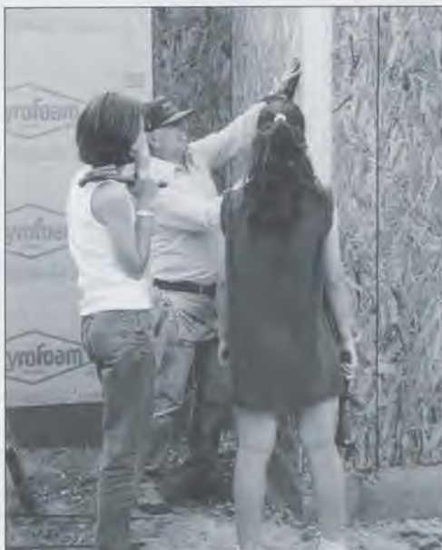
Ralph Harmon shows Ashleigh Cohen and Elizabeth Hutchinson how to nail up the particle board.
