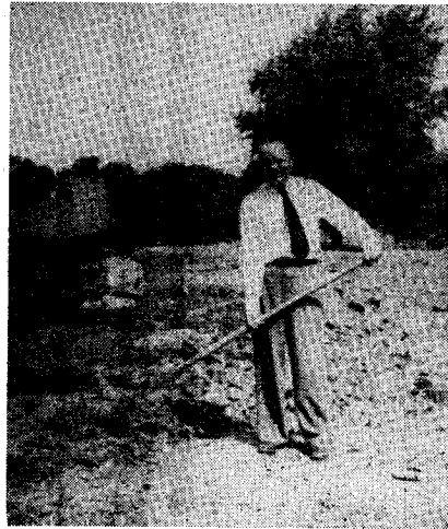
The London, Kentucky, pastor, J. D. Dobbs is shown in the picture breaking ground for the new London church. It is now in the process of building, and we believe the brethren and sisters there will be amply paid for the efforts put forth to bring about this splendid monument for the Lord in these last days.
