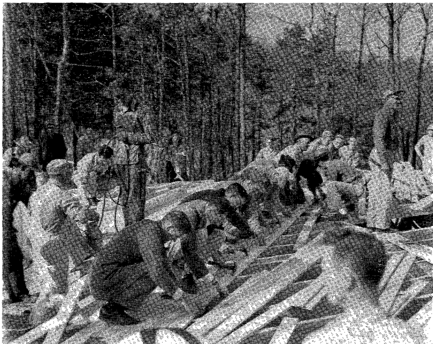
The men had a mind to work. At 8:50 A.M. they were already putting down the sub-flooring.
