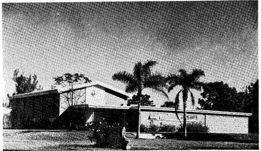
The Melbourne church showing new addition at extreme right.
