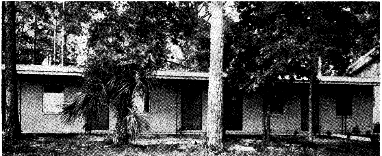
New educational unit in Cocoa, Florida. Four children's division Sabbath School rooms are here provided for. The building is situated behind the church, facing a side street.
