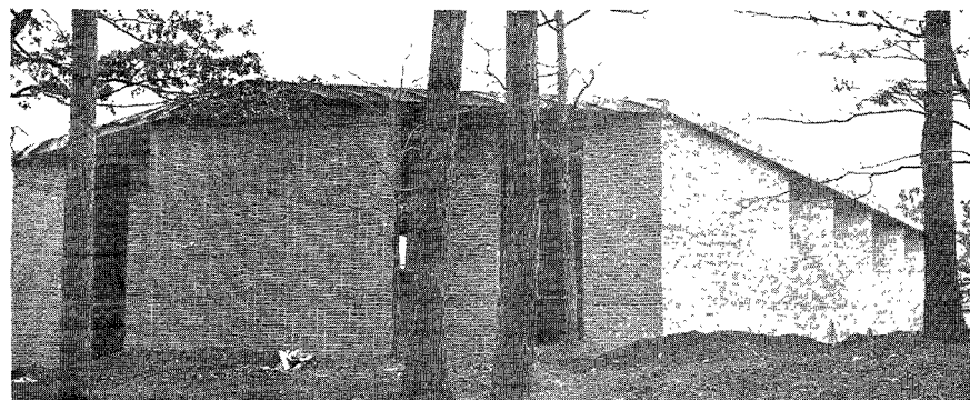
The chapel at the academy is now ready for finishing. The doors and windows will soon go in.
