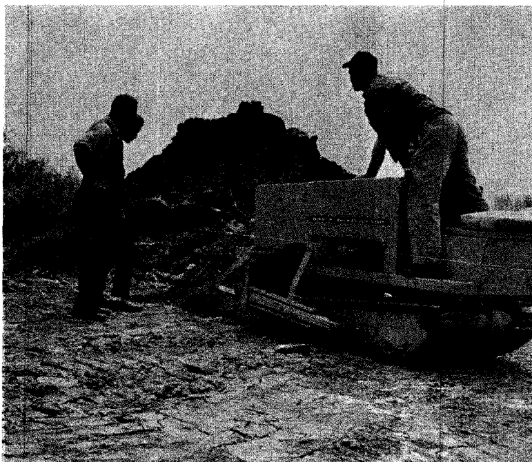
Construction work is just starting on a new apartment building. Students will be working in many of the building projects.
