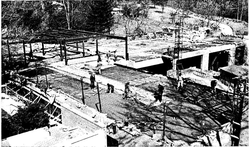
FLETCHER, NORTH CAROLINA — Construction on the new addition to the Mountain Sanitarium and Hospital is progressing on schedule. The new section will give an extra fifty beds for extended-care patients at a cost of $900,000. Opening date has been set for October, 1969.
