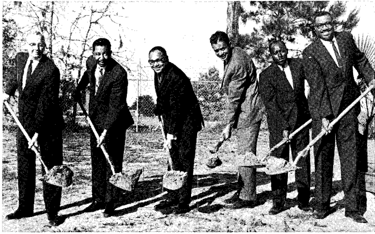
JACKSONVILLE, FLORIDA — Sunday, May 4, 1969, was a happy day for the Ephesus Jacksonville church—ground was broken for a new 600-seat capacity church building. From left, W. J. Keith, pastor of the Silver Street SDA Church; E. M. Johnson, city councilman; Harold Gibson, speaker for the occasion; W. S. Banfield, conference president; J. N. Williams, local elder; and R. B. Hairston, pastor of the church.
