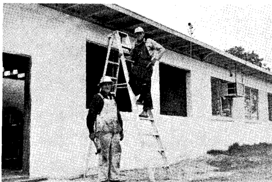
PANAMA CITY, FLORIDA — Enrollment in the Panama City elementary school jumped from 23 last year to 46 this year. The school plant has been doubled in size in recent months. Alex Brown and G. A. Huse have donated their time and led out with the construction. C. W. Reed is the pastor of the church.
