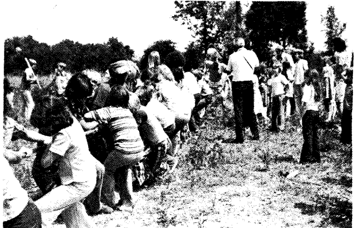
Instead of the usual pick and shovel, a turning plow, pulled by students, was used to break ground for the new Madison, Tennessee, elementary school. The 90 by 152-foot building will contain eight classrooms. Construction is expected to be completed in time for school this fall.
