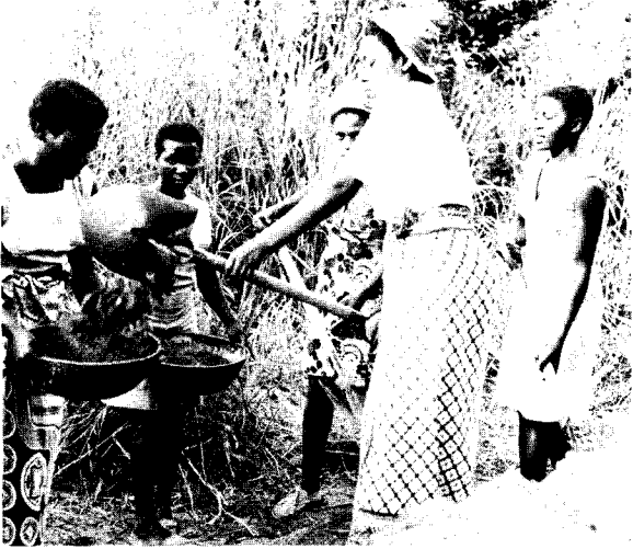
These young Parane women carried this sand from the river bank to the building site where it was mixed and made into bricks for the Parane Secondary School's science laboratory, built in 1977, in the Pare Mountains of Tanzania. This quarter's 13th Sabbath offering will help to build a new dormitory there. The students have had to live in the classrooms because of insufficient living space in the present dormitories.
