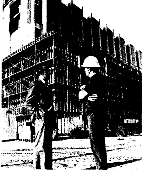
Mardian Blair, president of Florida Hospital, and Larry Arnold, project foreman for H. J. High Construction Company, estimate that construction on the new patient areas at Florida Hospital/Altamonte should be completed some time this spring. The addition of 86 medical and surgical beds will bring the total to 225.
