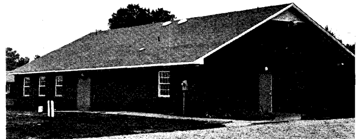
A new church school building was constructed in Raleigh, North Carolina, during the summer of 1982. Pastor Wayne Owen, assisted by his father and members of the church, poured the concrete, laid the bricks, and did most of the construction work themselves. The building has three classrooms and a small auxiliary room. Future plans call for the addition of a gymnasium-auditorium. Total enrollment is 32. Grades 1-8 are taught by Janet Griffin and Dean Flint. Cheryl Goldston operates a kindergarten. The school is located on several acres of land where the new Raleigh church building will also be constructed when plans are completed. The present pastor is Charles Hindman.
