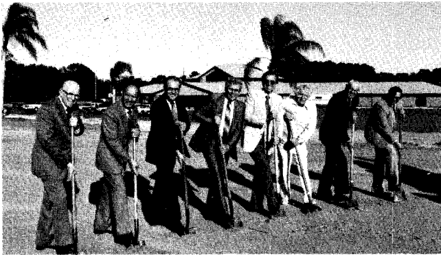
"Digging in" for Maranatha Flights International. This octet of smiling faces with busy shovels met to break ground for the Maranatha Living Center on December 7, 1983. This retirement center is being built adjacent to the recently completed New Port Richey, Florida, church (in the background) to provide financial support for MFI. For further information write to Box A, Berrien Springs, MI 49103. Pictured are: R. H. Pierson, former General Conference president (left); H. J. Carubba, Florida Conference president; J. P. Rogers, Florida Conference treasurer; John Freeman, MFI president; John Bullock, MFI Living Center chairman; Wayne Schaffer, George Vandenberg, and Roger Hatch.
