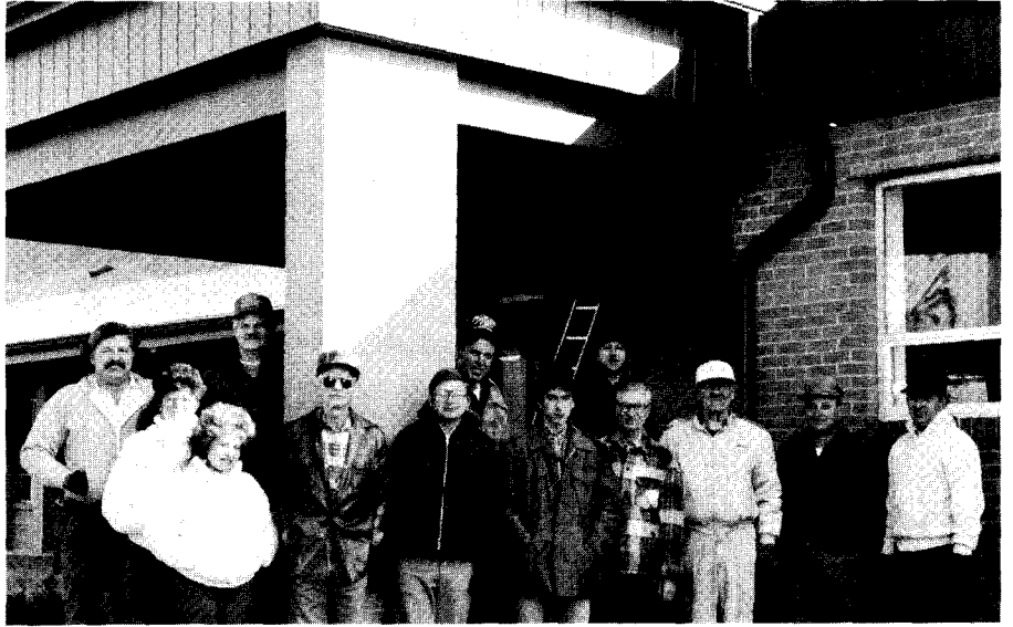
Pictured above are laymen from the Covington, Ky., church who devoted eight Sundays to improve the appearance of their church and school. Dave Fleissner (left), volunteered to supervise this project. The installation of new siding and eaves was completed. This eliminates all future painting and repair. The work was completed for $6,000 less than had been quoted on the contract bid.
