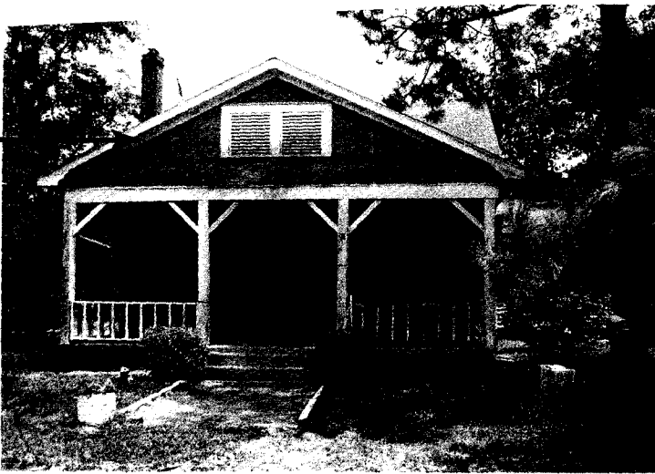
The brown shadow across the attic air vents gives an idea of the water level during the flood which swept away coffins from grave sites, pets from roof tops, and people out of trees.
