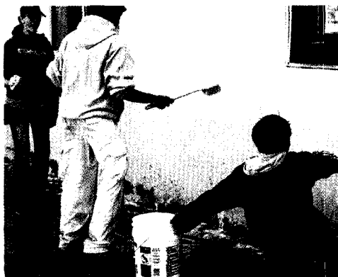
The goal was to prepare the walls for painting.
