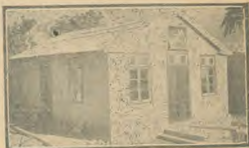
Pictured above is the recently completed neat little church building in Jericho, West Jamaica. It is a real credit to the district. During 1948 we hope to complete many more such representative edifices.
